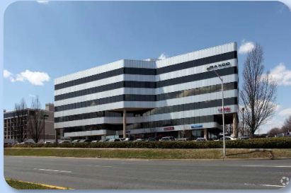
6 Montgomery Village Avenue
